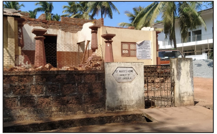
St. Mary's Home Goa Architect Mr. Jose L Noronha Contractor- Mr. Jose Mario
